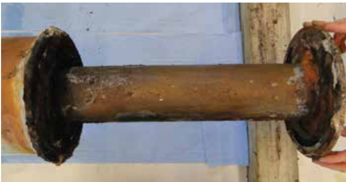
Figure 4. Image of the lower, underside, of the pipe
